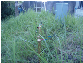
Fig. 4 Installation of detectors into ground
